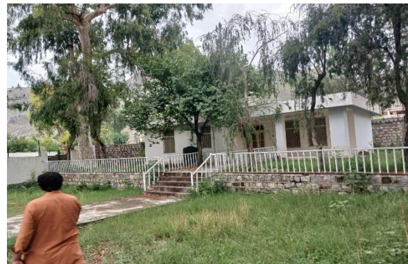
A view of the existing rest house building at the proposed residential complex site.
