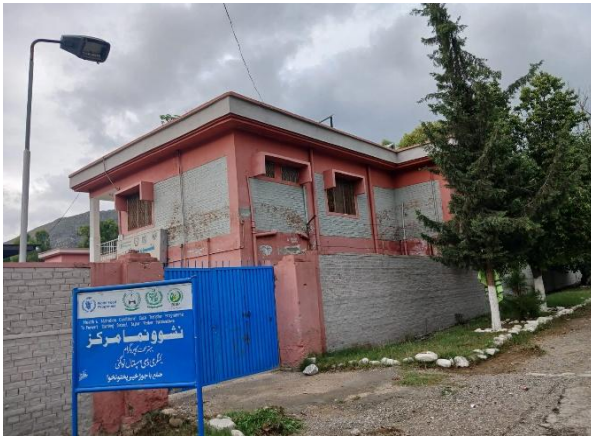
A view of the Tehsil Headquarters Hospital.
