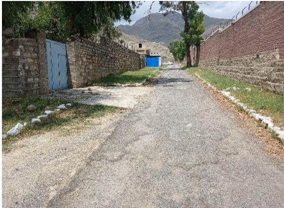
A view of the existing building of the rest house at the proposed Residential Complex Site (at the right) and quarters at left
