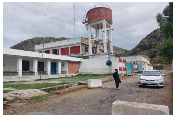
A view of the Rescue 1122 Office.
